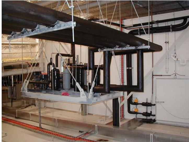
Fig. 5. R744 (CO<sub>2</sub>) Condensing Unit installed in ceiling cavity
