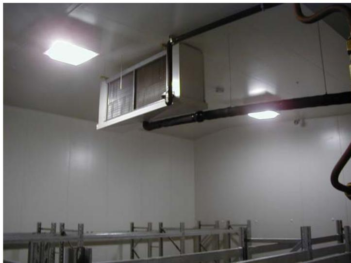
Fig. 6. Finned air cooler suitable for R744 (CO<sub>2</sub>) refrigerant and installed in the cold store
